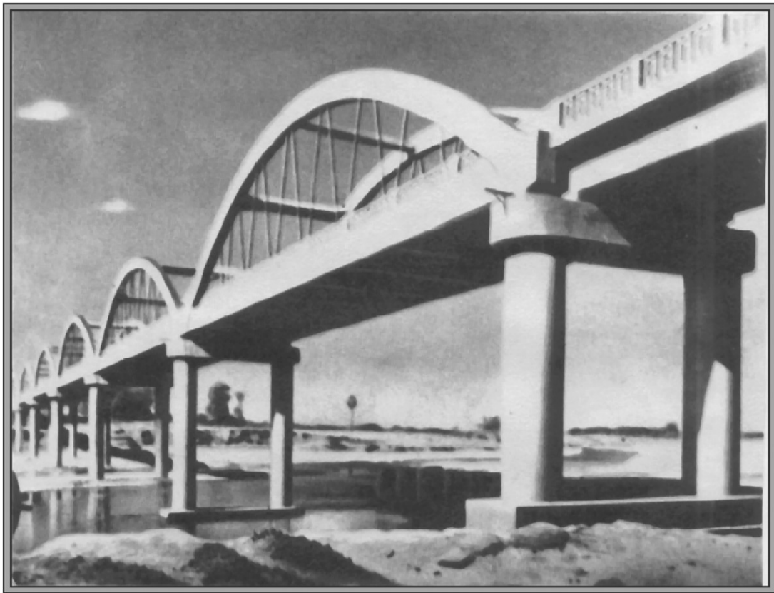
Fig. 1.5: Bow string girder bridge
